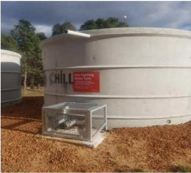
Strategic 47,000 Litre Concrete Tank & Protected Fittings
