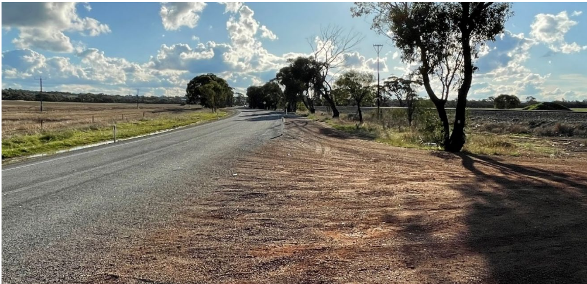
Figure 4: Northam – York Road looking northwest from existing level crossing
