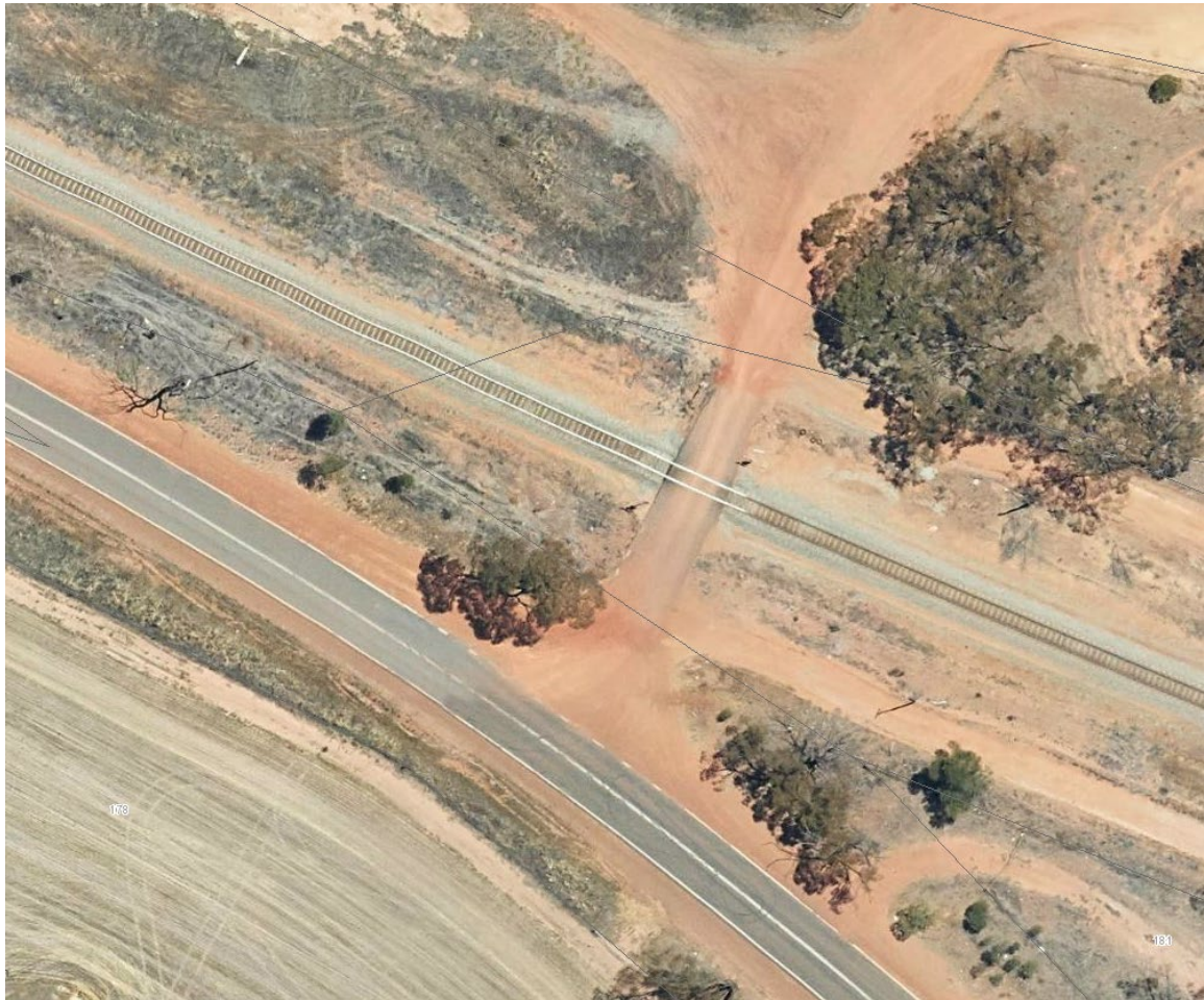
Figure 8: Northam – York Road and existing level crossing
