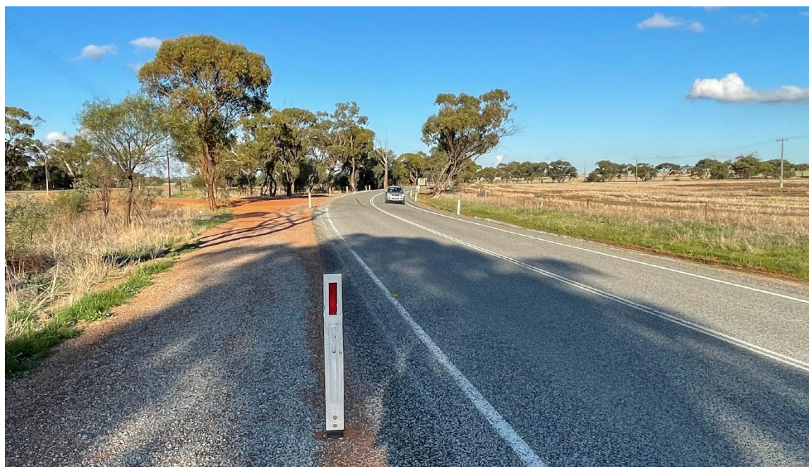
Figure 7: Northam – York Road looking southeast (level crossing to the left)
