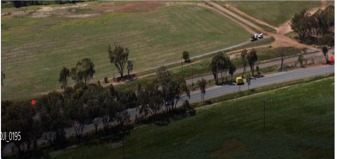
Figure 15 3D Drone Viewpoint From South Showing Site Access
