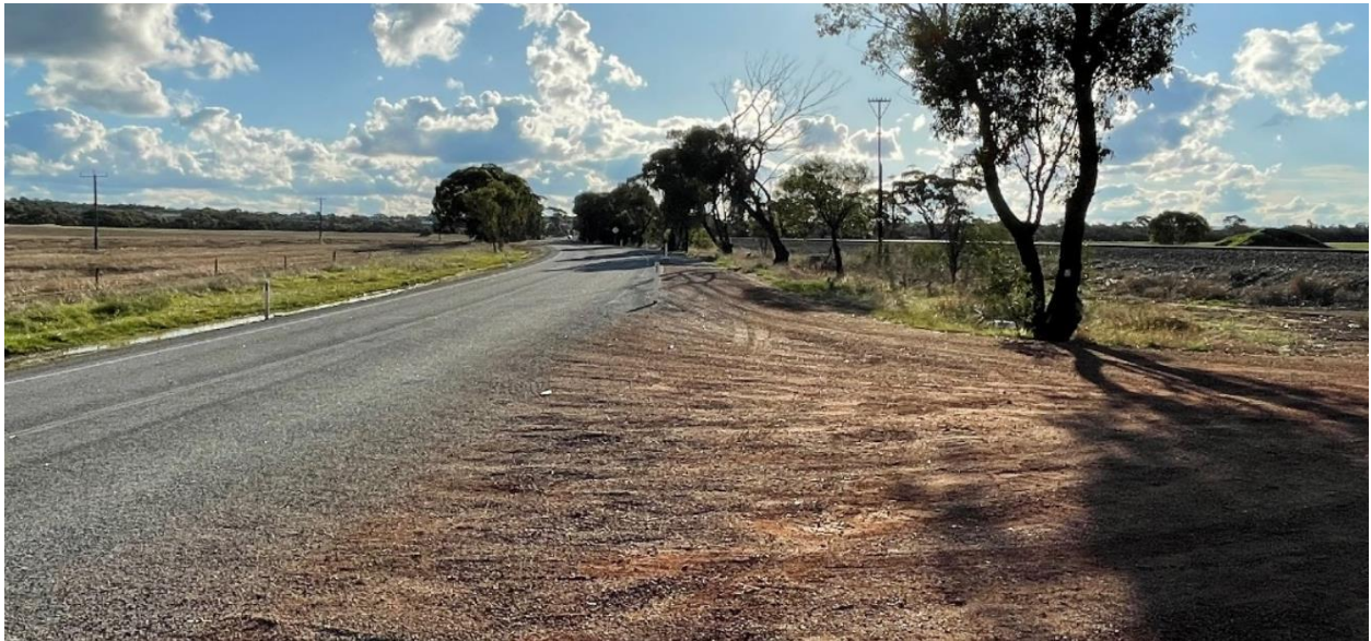
Figure 8: Northam-York Road Looking West
