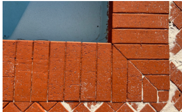
Unit paver header to back of kerb: Midland Heavy Duty Red, laid on edge
