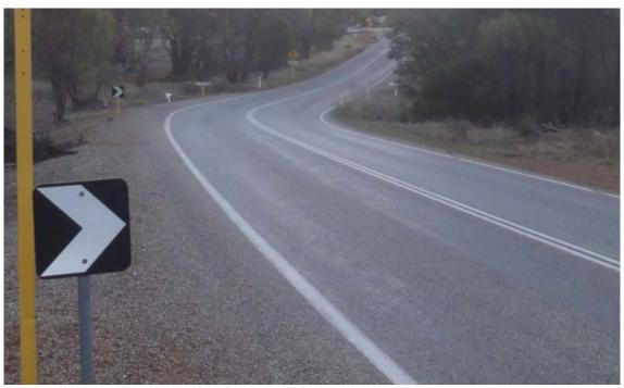
Finding 2.19 – Curved alignment markers – Incorrect and damaged signs present
