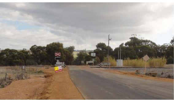
Finding 2.7 & 2.25 – Pavement markings missing removed from roadworks, and narrow approach seal 2.7m – Also note singled sided speed zone
