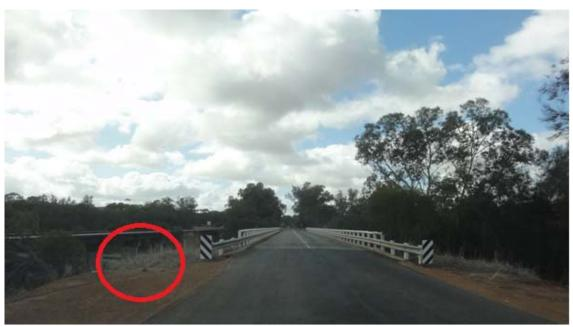
Finding 2.14 – Bridges – Barrier system length would not provide protection of errant vehicle
