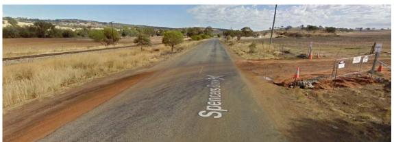
Finding 2.4 – Quarry Access – Evidence (old) of large vehicles using shoulder
