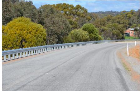
New guard rails near Mokine Road – centreline of the road to the guard rails is 4.4 metres.
