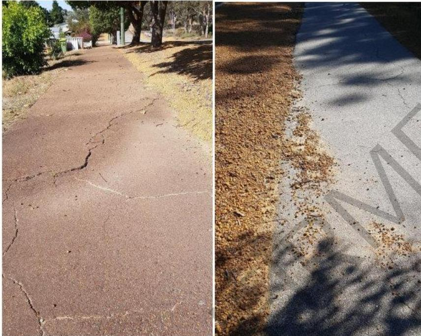
Photos 20 & 20a: Loose material and pavement defects along the path in Baker's Hill.
