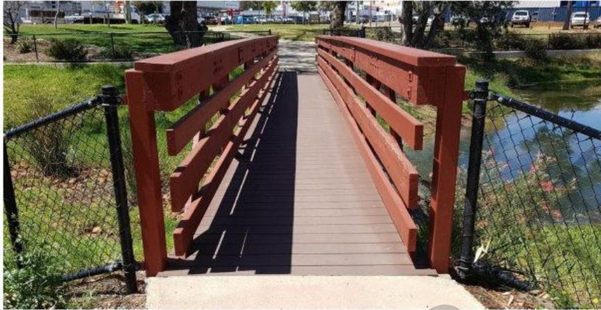
Photo 11: Narrow bridge with bike unfriendly parapets.
