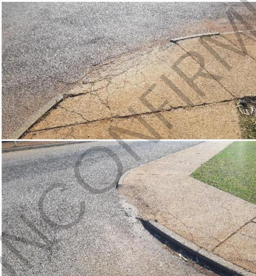
**Photos 13 & 13a:** These examples of sub-standard pedestrian ramps are in Wundowie.
