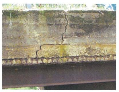
Photograph 11: Crack to concrete deck edge.
