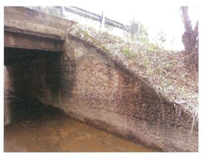
Photograph 6: Typical abutment (Abutment 2).
