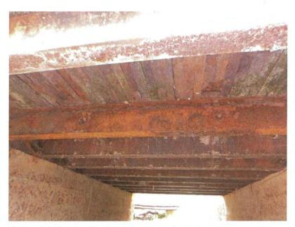
Photograph 5: Underside of bridge – note widespread corrosion to beams.
