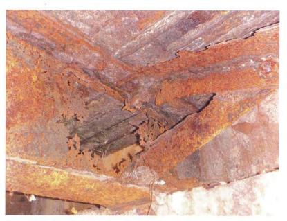
Photograph 7: Corrosion perforation to Abutment 1 end of Beam 9.
