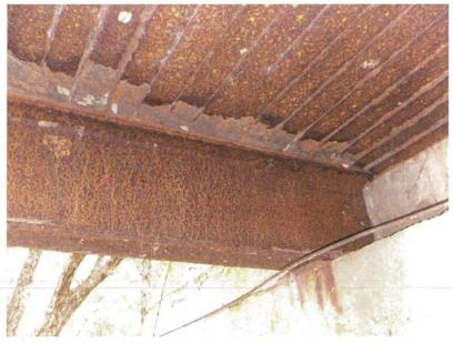
Photograph 10: Typical corrosion to beams and transverse beams.
