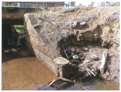
Photograph 14: Scour behind Abutment 1 Left Hand Side Wing Wall.
