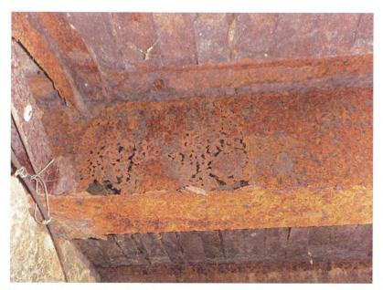
Photograph 8: Corrosion perforation to Abutment 2 end of Beam 9.
