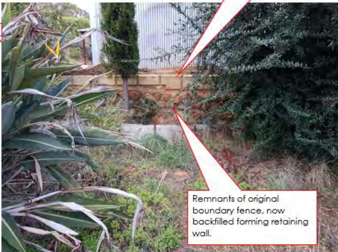
Remnants of original boundary fence, now backfilled forming retaining wall.
