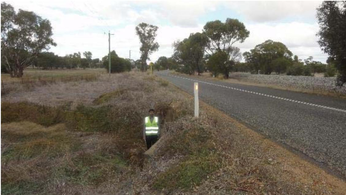
**Finding 2.9 – Safety issues around culvert – Tall culvert within clear zone with no warning or protection other than a single guidepost (that is typical treatment of the road without culvert hazards)**
