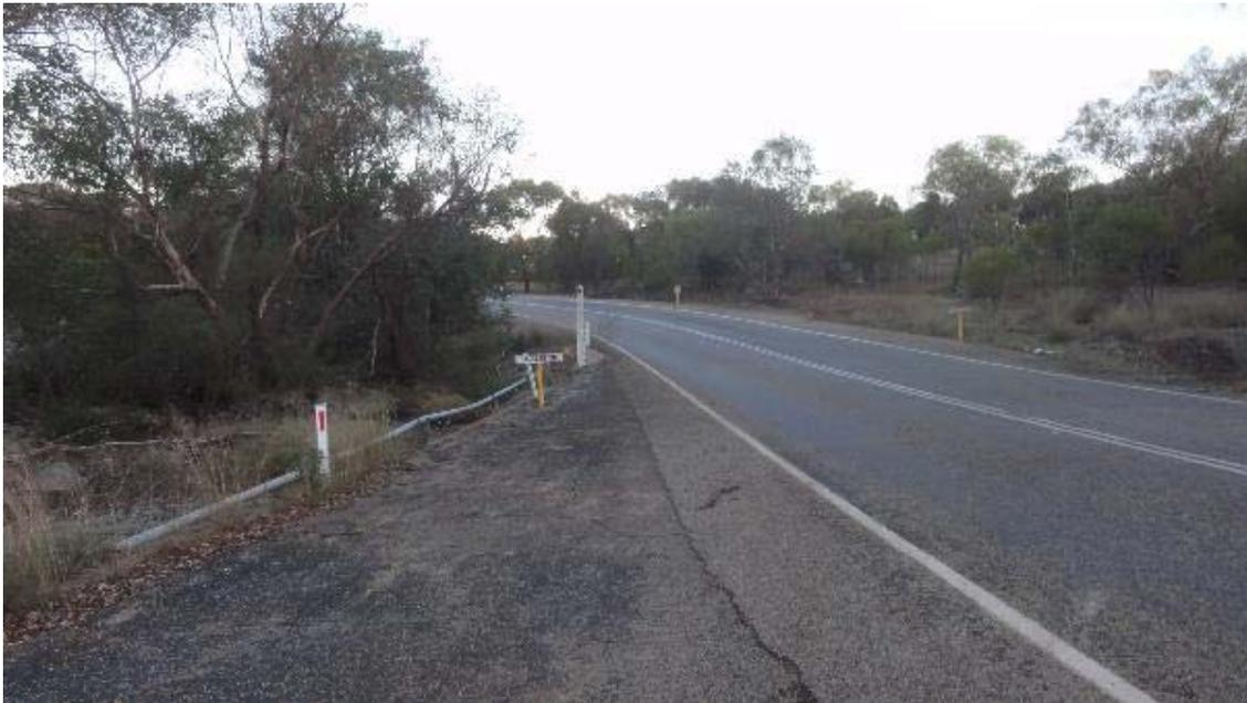
**Finding 2.9 – Safety issues around culvert – Tall culvert within clear zone with no warning or protection**
