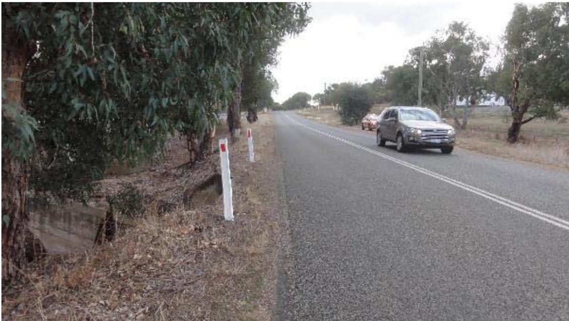
**Finding 2.9 – Safety issues around culvert –Culvert within clear zone with no protection**
