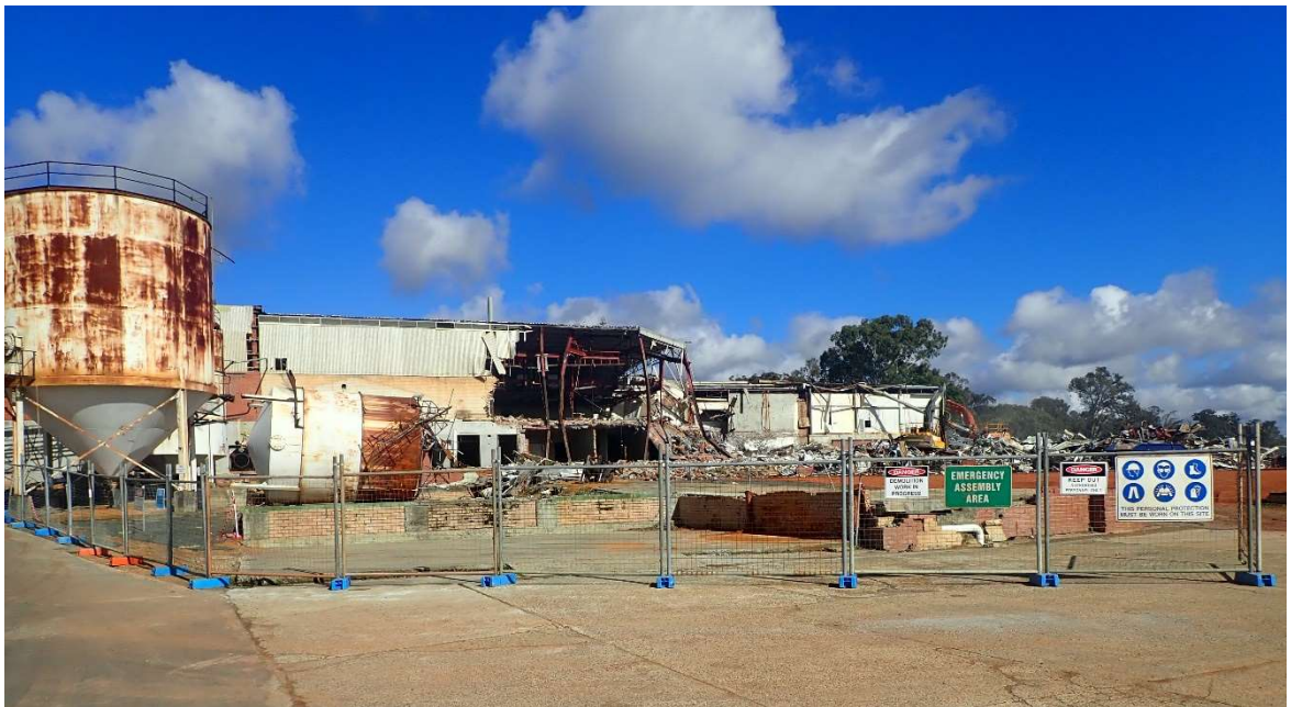
Figure 2 Demolition in Progress
