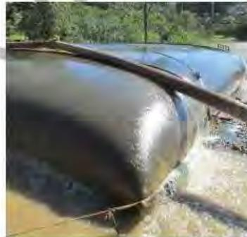
**Figure 5-3: Dewatering of a Geotube**
