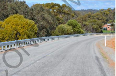
New guard rails near Mokine Road – centreline of the road to the guard rails is 4.4 metres.
