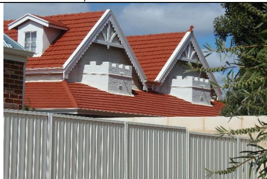
Gables with battlemented parapets Source: Stephen Carrick Architects October 2021
