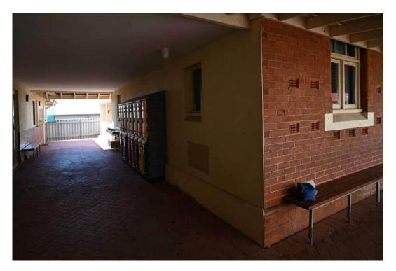
Photograph 5 Western corner of D&T building under awning. Note awning cutting across openings. Art and Home Economics building to the left. *Griffiths Architects Aug 2024*
