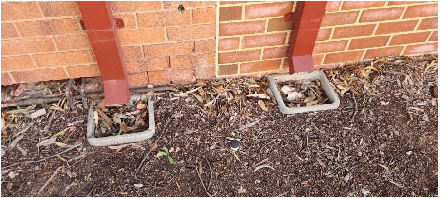
Photograph 9: Downpipes discharging into concrete drain boxes: note leaves clogging drains
