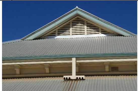
Ventillation gablet Source: Stephen Carrick Architects September 2021
