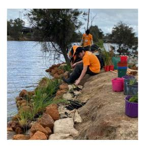
Curtin University. The project involved moving 10 tonnes of rock, soil and mulch by hand with the use of a barge over to the island. Rock and sandbags filled with soil medium were used to stabilise the perimeter and build up vegetation bed areas so that native tube stock could be planted to improve the degraded condition of the island.
