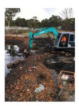
Completion of base earthwork level. this is about 600mm lower than the invert level of the upstream culvert
