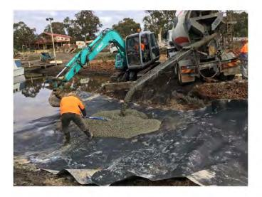
f. Completion of concrete work. The finish top concrete level is about 400mm lower than the invert levels of upstream culverts
