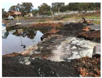
e. Construct 200mm thick 32MPa concrete spillway
