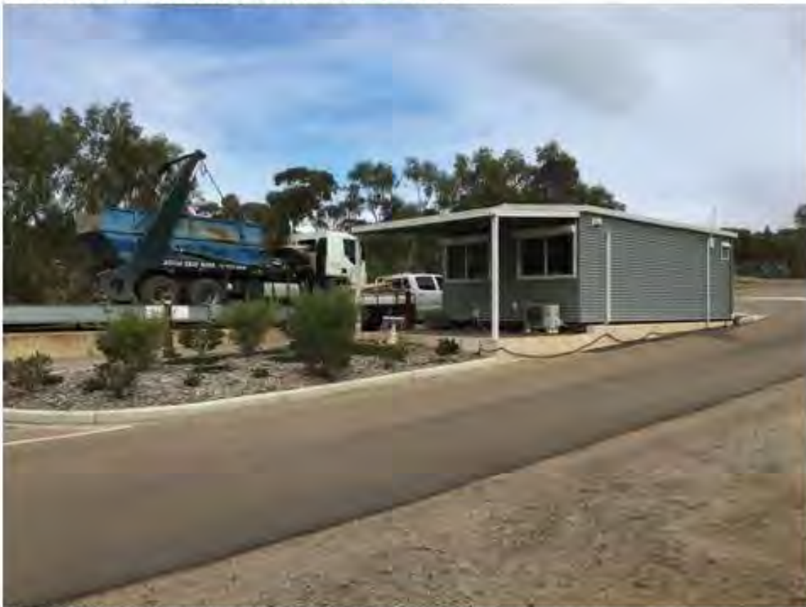
Old Quarry Road Site Entrances – Weighbridge and Gatehouse
