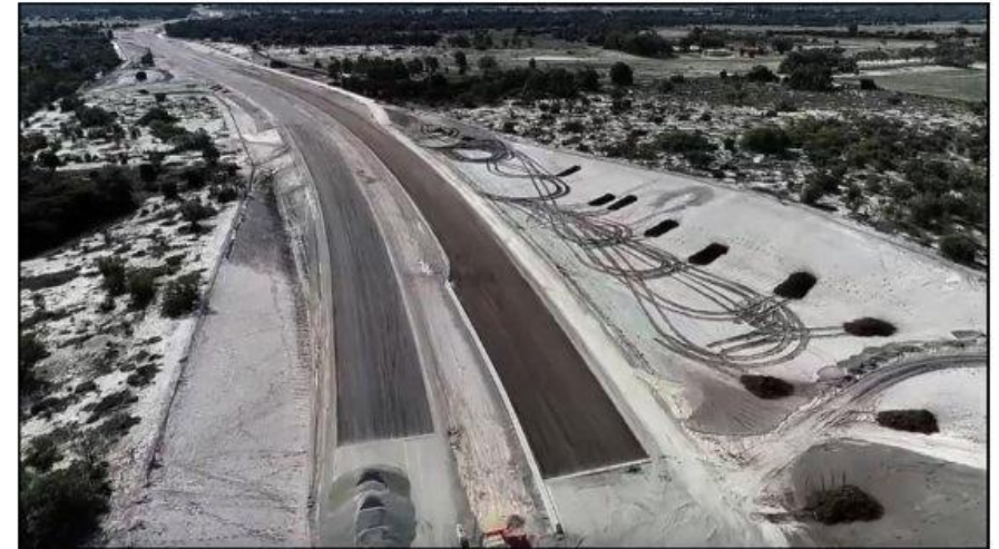
North-link project construction
