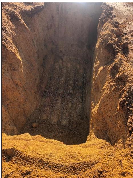
Photo 1: Excavation showing gravel, clay and laterite
