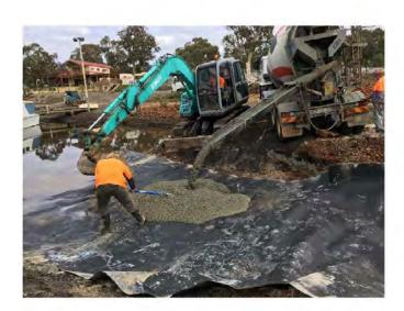
f. Completion of concrete work. The finish top concrete level is about 400mm lower than the invert levels of upstream culverts
