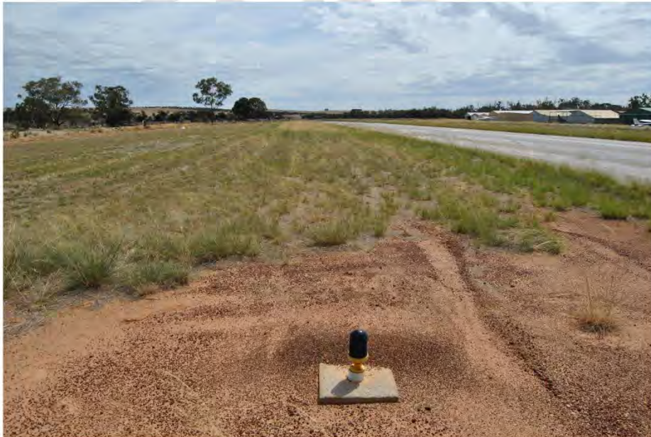
Concrete blocks should be flush with the surrounding area on the Runway Strip.
