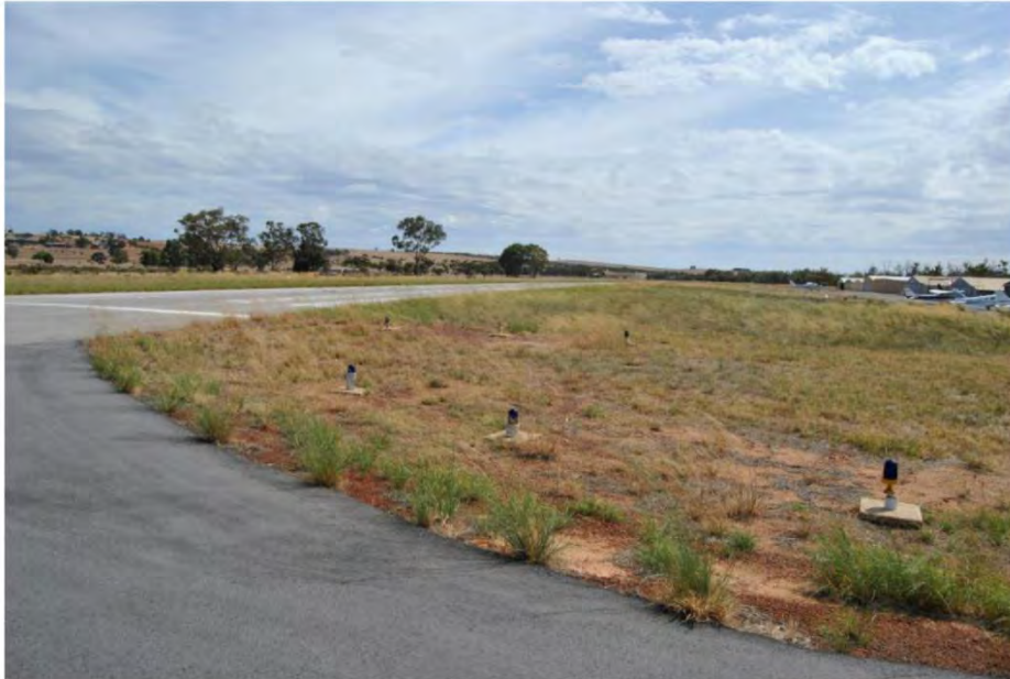
View facing north-west from the southern taxiway. Runway threshold and taxiway edge lighting.
