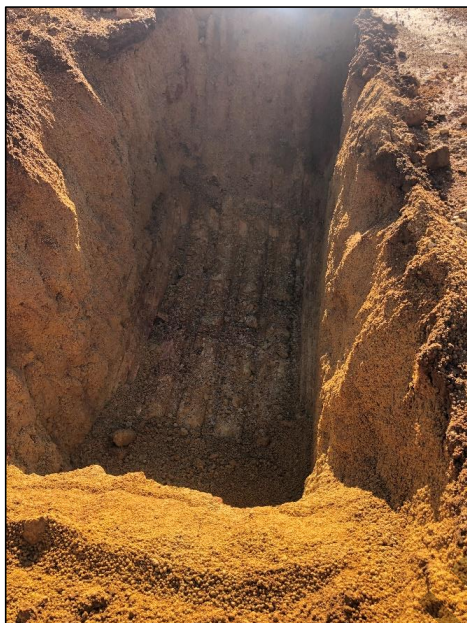
Photo 1: Excavation showing gravel, clay and laterite
