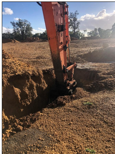
Photo 2: Excavated gravel pit – typical depth
