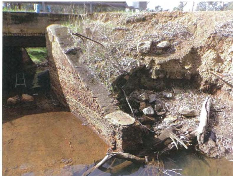
Photograph 14: Scour behind Abutment 1 Left Hand Side Wing Wall.
