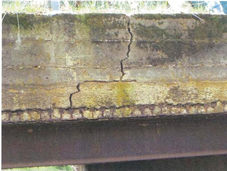
Photograph 11: Crack to concrete deck edge.
