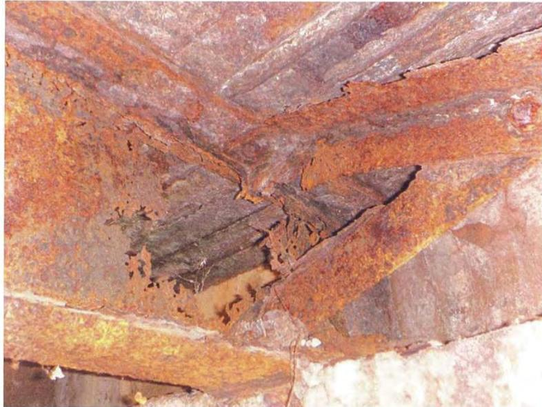
Photograph 7: Corrosion perforation to Abutment 1 end of Beam 9.
