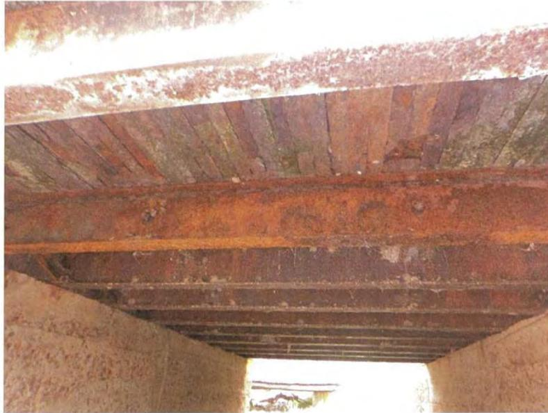
Photograph 5: Underside of bridge – note widespread corrosion to beams.
