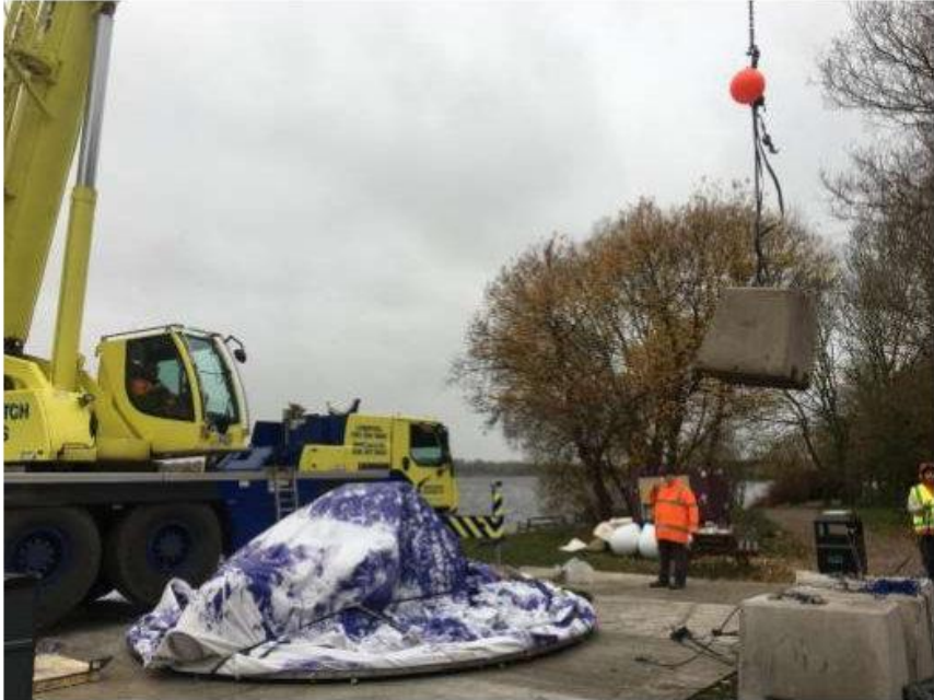
Concrete is craned into position and location marked with marker buoys.
