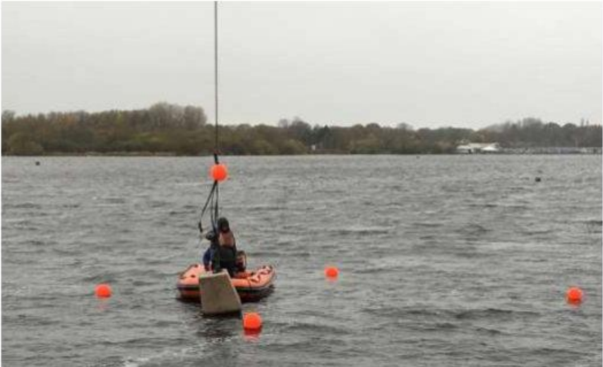
Alternatively, the concrete blocks can be lowered in from a barge.
