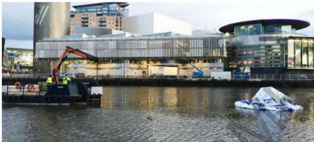
Alternatively, the concrete mooring can be placed into the water with a barge.
