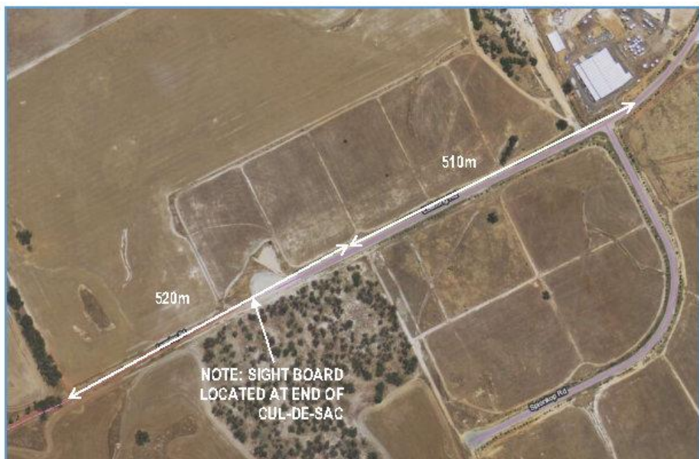
Figure 12: Site Access SISD
