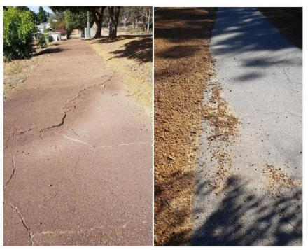
Photos 20 & 20a: Loose material and pavement defects along the path in Baker's Hill.
