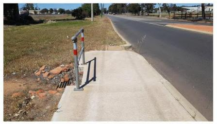
Photo 14: This barrier does not effectively protect road users from the grating, but does present a hazard.
