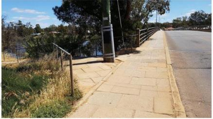
Photo 15: Poor barriers that could cause injury, especially to cyclists.
