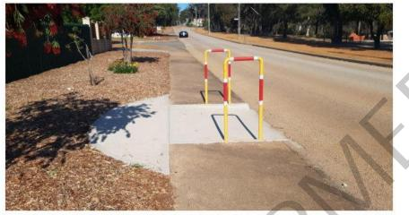
Photo 24: Not all cycling facilities are installed to standard.
