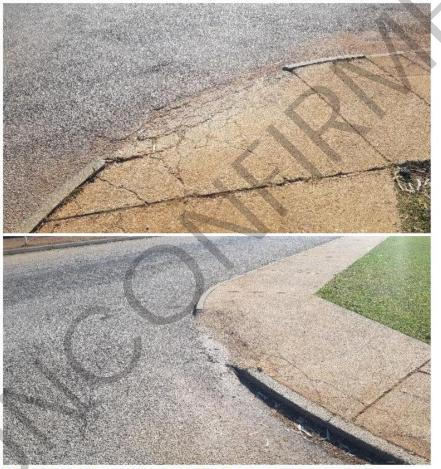
Photos 13 & 13a: These examples of sub-standard pedestrian ramps are in Wundowie.
