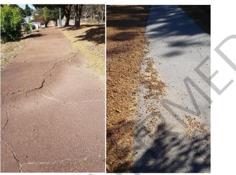
Photos 20 & 20a: Loose material and pavement defects along the path in Baker's Hill.
