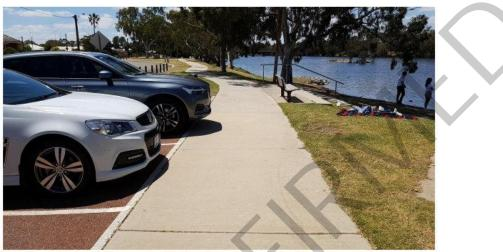
Photo 18: Lack of wheel stops means parked cars become a hazard to path users.
