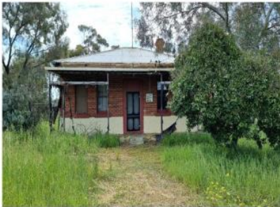
At commencement of Lease
