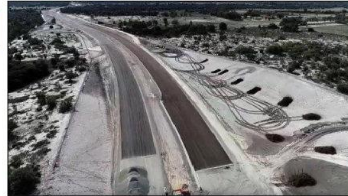
North-link project construction
