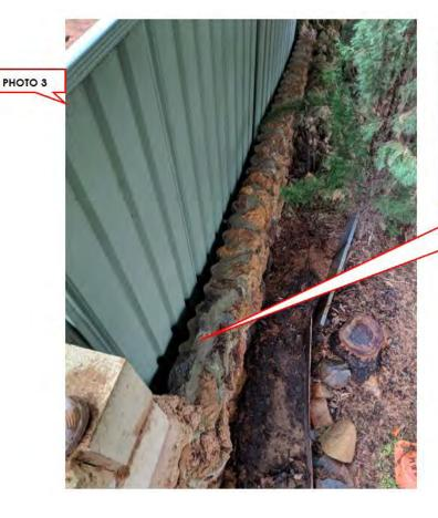
Super 6 fence panel's cladded with mortared rocks on the Eastern Side (typical of entire original fence)
