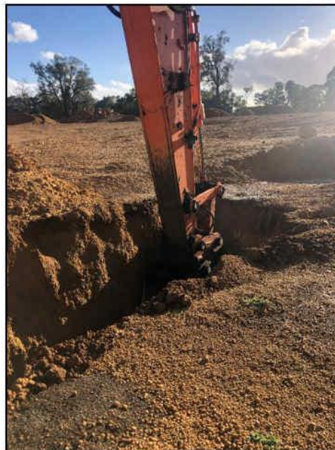
Photo 2: Excavated gravel pit – typical depth
