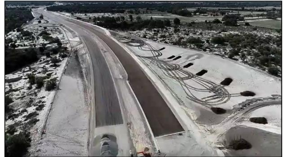
North-link project construction
