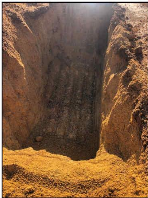
Photo 1: Excavation showing gravel, clay and laterite
