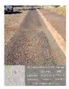
Existing issues: Pavement Failure & Rutting, Pot Holes
