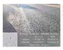
Existing issues: Isolated Pavement Failure & Rutting
