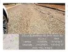
Existing issues: Stripping, Cracking and Surface
