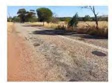
Existing issues: Surface Age, pavement failure, potholes, cracking
