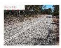
Existing issues: Very Heavy Stripping and cracking
