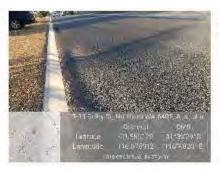
Existing issues: Isolated Pavement Failure & Rutting
