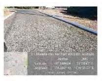
Existing issues: Stripping & Cracking
