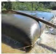
Figure 5-3: Dewatering of a Geotube
