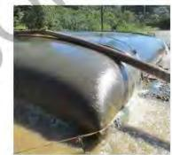
Figure 5-3: Dewatering of a Geotube
