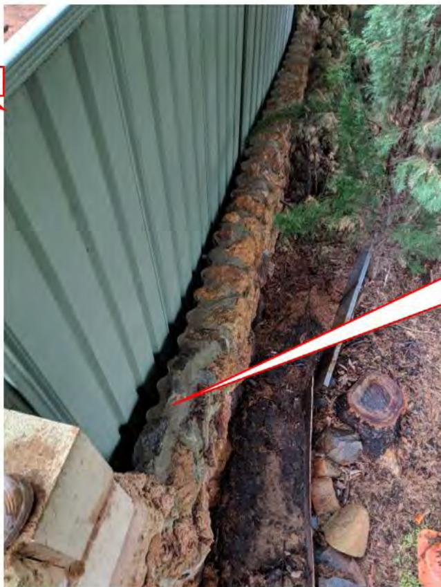
Super 6 fence panel's cladded with mortared rocks on the Eastern Side (typical of entire original fence)
