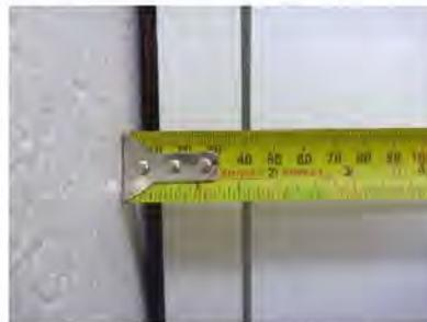
*Reduced latch clearance (40mm)
