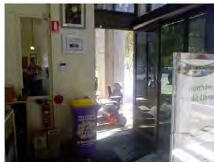
Narrow door opening (695mm) with high door controls (1265mm)
