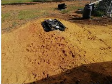
Septic tank fully covered
