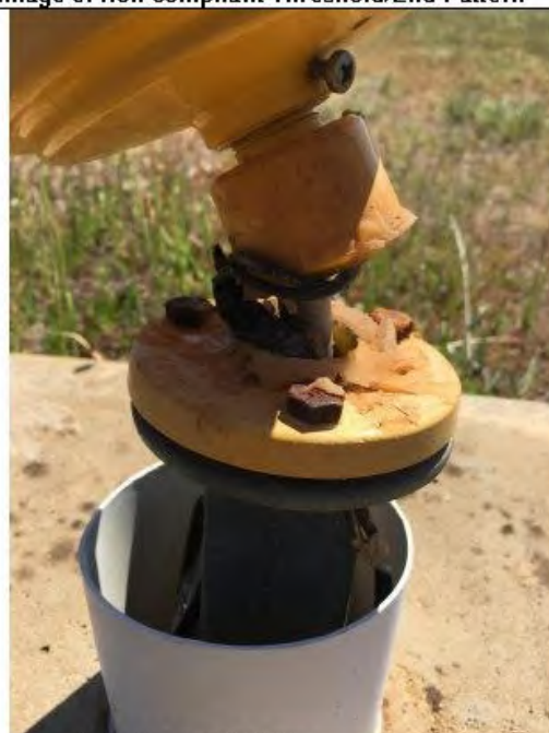
Image 8: Broken Light Fitting
