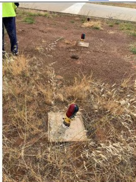
Image 6: Non compliant Threshold/End Pattern
