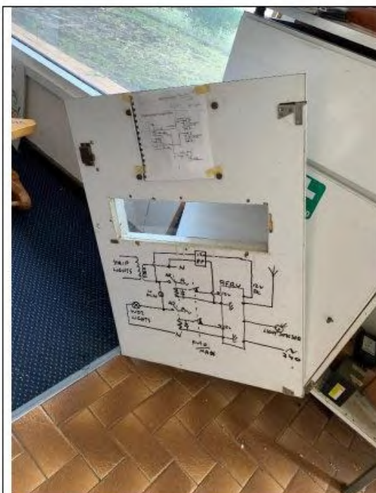
Image 5: Control Panel Door-Circuit Diagram
