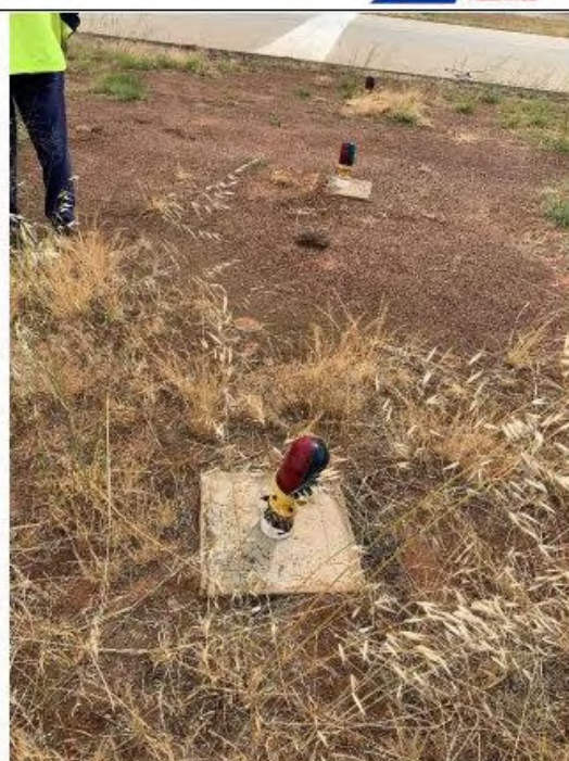
Image 6: Non compliant Threshold/End Pattern
