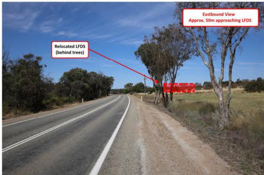
Figure 4-1 Great Eastern Highway View Eastbound
