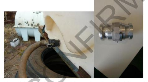
Above: a Typical "Farmer Unit" showing existing connector and hose which with the use of a BIC to Camlock adaptor could connect to the new hydrant outlet.
