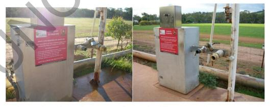
Toodyay Stand pipe showing their conversion from overhead fill to Hydrant style connection. Note this is also a public access point hence the additional connections.
