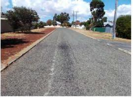
Road Hierarchy: LOCAL ROAD RAV Route (Y/N): No Bus Route (Y/N): No Shire Focus (RRG): No Trigger source: RAMM Ranking: 62 Asphalt Overlay Proposed Works: Associated Works: remove / replace kerbing \$51,058 Treatment Cost:
