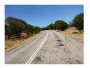
Road Hierarchy: **REGIONAL DISTRIBUTOR** RAV Route (Y/N): YES Bus Route (Y/N): YES Shire Focus (RRG): YES Trigger source: RAMM Ranking: 28 Proposed Works: Widen and seal for 8.3 m road Cement stabilise road failures. Associated Works: \$349,064 Treatment Cost:
