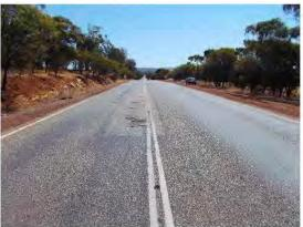
Road Hierarchy: **Regional Distributor** RAV Route (Y/N): Yes Bus Route (Y/N): Yes Shire Focus (RRG): No Trigger source: RAMM Ranking: 23 Proposed Works: Mill & Replace Associated Works: Nil Treatment Cost: \$160,351
