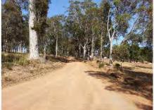
ICS Ranking: N/A Proposed Works: Regravel with V Drain. Drains & driveway culverts Associated Works: Treatment cost : \$409,540
