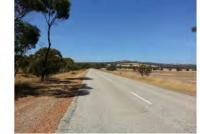
Road Hierarchy: **REGIONAL DISTRIBUTOR** RAV Route (Y/N): YES Bus Route (Y/N): YES Shire Focus (RRG): Trigger source: RAMM Ranking: 448 Proposed Works: Widening to 8.3m and Spray seal Associated Works: \$203,391 Treatment cost:
