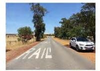
Road Hierarchy: **REGIONAL DISTRIBUTOR** RAV Route (Y/N): YES Bus Route (Y/N): YES Shire Focus (RRG): Black Spot Trigger source: RAMM Ranking: priority ranking 44 Proposed Works: Road widening to 7m Associated Works: Culvert extension Treatment cost: \$141,672
