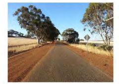
Road Hierarchy: RAV Route (Y/N): Bus Route (Y/N): Shire Focus (RRG): Trigger source: Ranking: Proposed Works: Associated Works: Treatment Cost: LOCAL DISTRIBUTOR YES YES RAMM, Complaints from residents 199 Widening to 7m and Spray seal Drainage & Culvert extensions \$233,396
