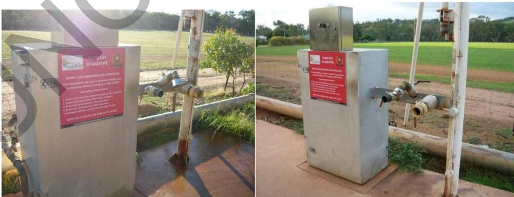
Toodyay Stand pipe showing their conversion from overhead fill to Hydrant style connection. Note this is also a public access point hence the additional connections.
